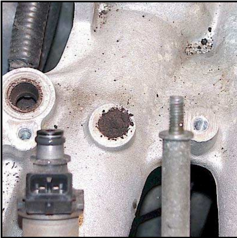
Here is a close-up shot of a clogged EGR port.
